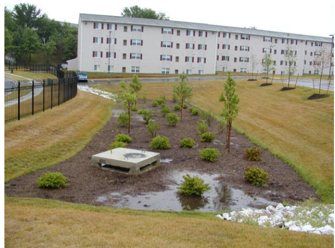
Runoff from parking lot entering bioretention facility in Maryland.
